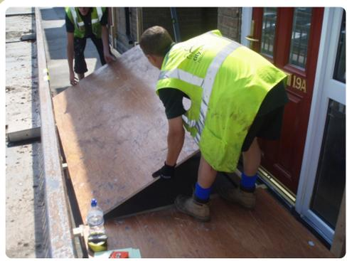
Temporary panels are laid on the framework which can be lifted and replaced to allow the flooring to be laid
