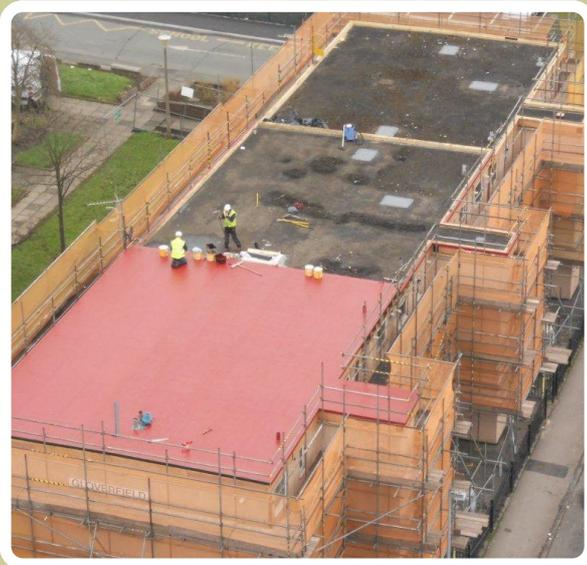
The flat roofing system was designed by Sika and consisted of 130mm of PIR insulation board covered by a decothane roof membrane.
